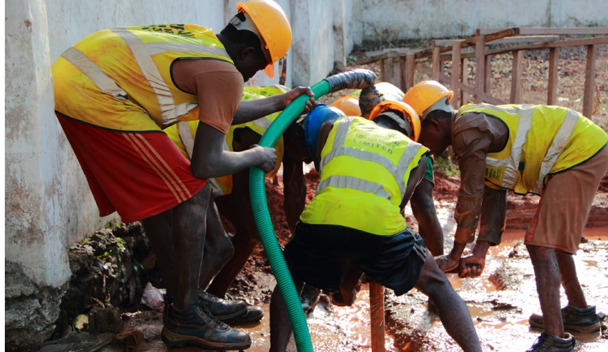
Manual drilling in Lagos, Nigeria
